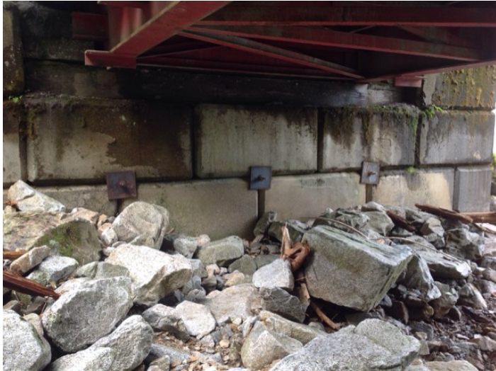
Left Bank Abutment when facing downstream
