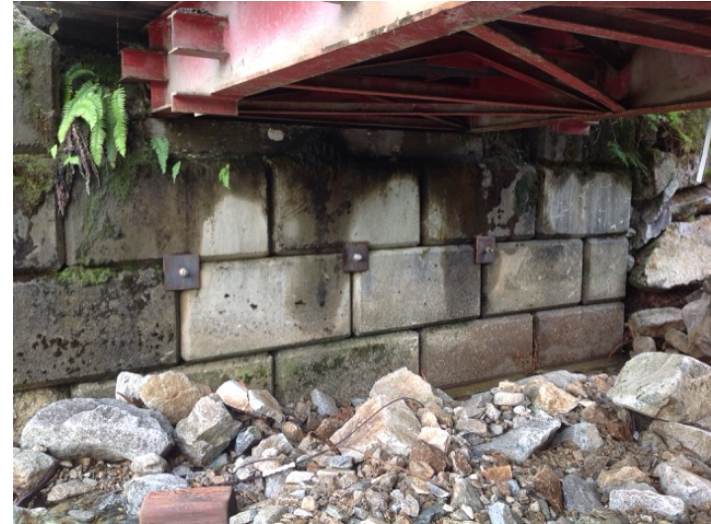
Right Bank Abutment when facing downstream
